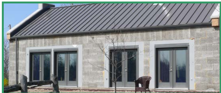
Training Centre—under construction.
